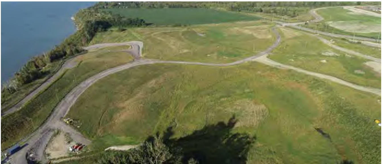
Port Granby Long Term Waste Management Facility - Over 1.3 million tonnes of waste excavated from the Lake Ontario shoreline in Southeast Clarington is now safely stored in the engineered, aboveground storage mound that was capped and closed in fall 2021.
